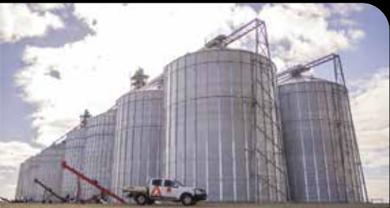
SITE CONSTRUCTED SILOS
