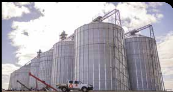
SITE CONSTRUCTED SILOS
